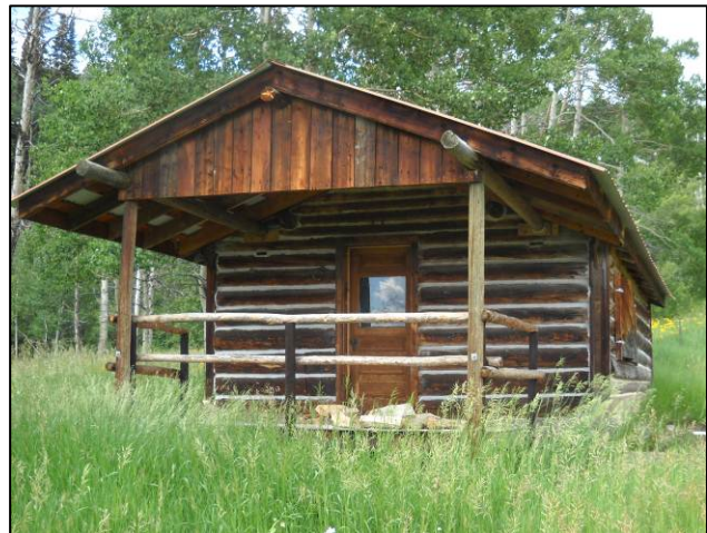
Figure 6. A homestead is located on the Property and includes three buildings.
